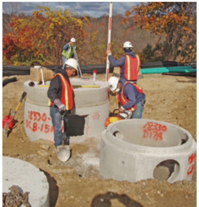
Masterson crew works on utility system manholes.
