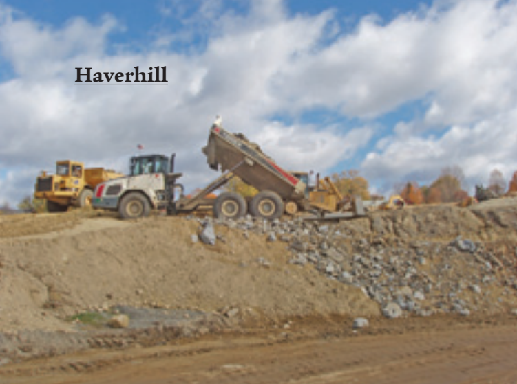
A Terex truck discharges shot rock while a CAT truck passes with another load of rock.
