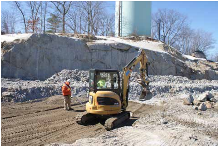
A CAT mini-excavator cleans up area near water tower.
