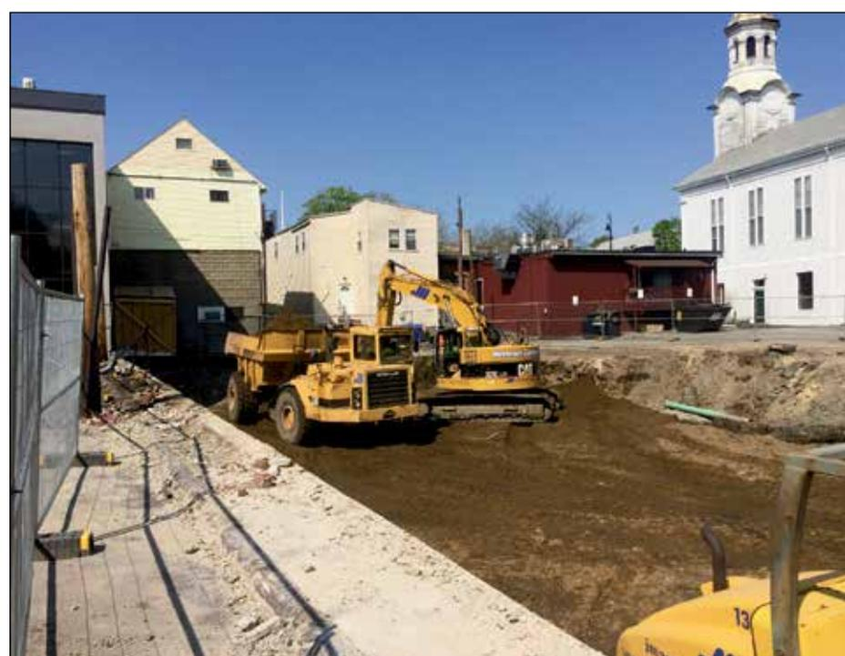
A Caterpillar 321 Excavator works with a Caterpillar D25 off-highway truck to backfill the site of a building razed by New Hampshire Demolition.
