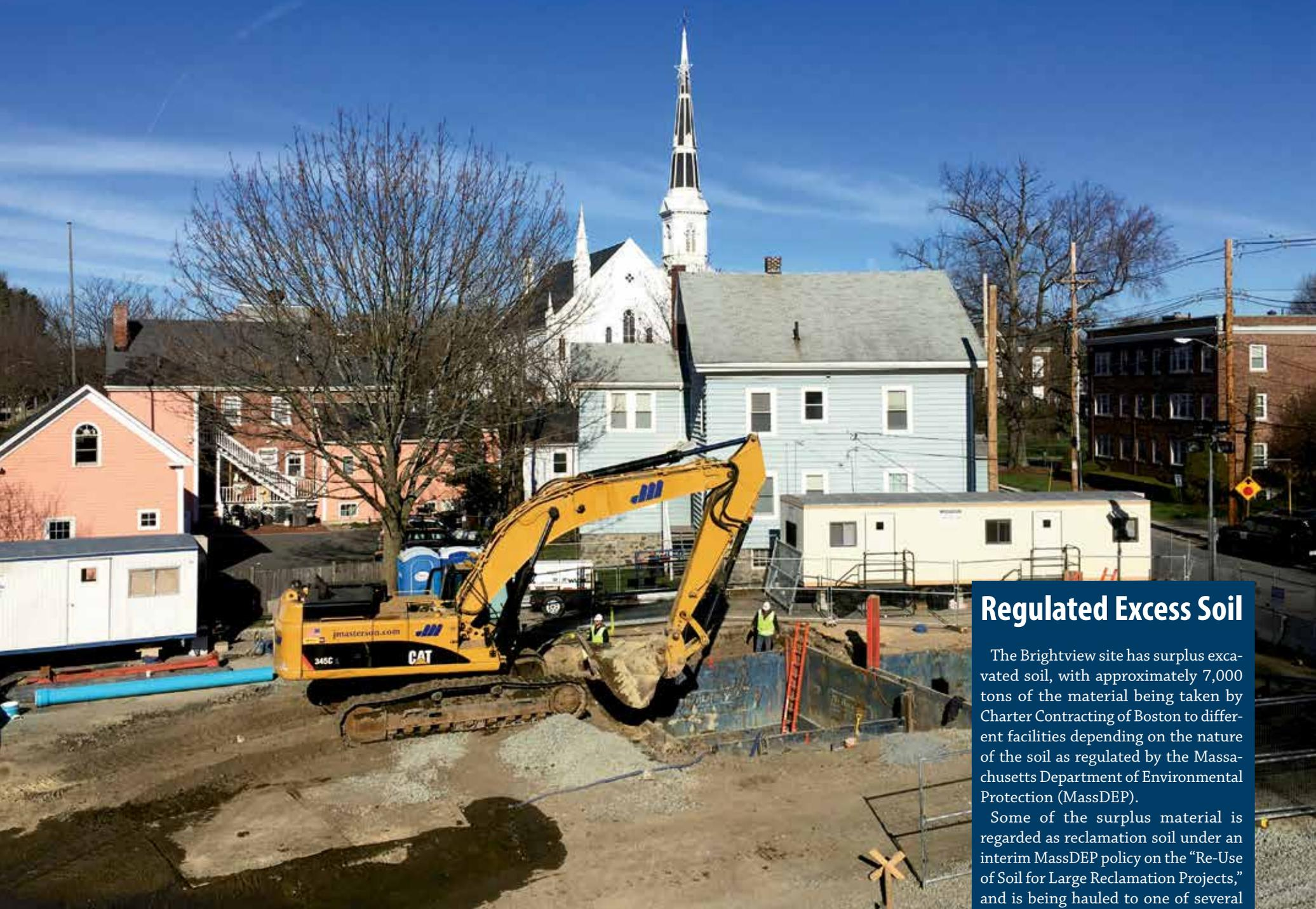
A Caterpillar 345 excavates for deep 12-inch PVC sewer within two end-to-end Mabey Slide Rail installations.
