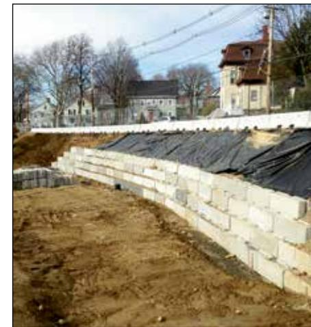
Masterson built battered earth retention wall with 3,000-pound blocks provided by MacLellan Concrete Co., while Shea Concrete highway barriers line edge of adjacent street for safety.
